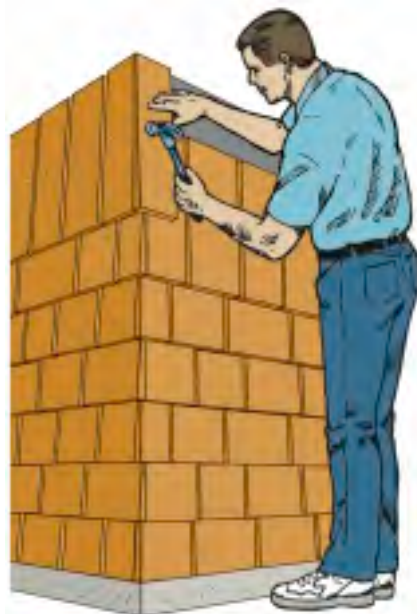
Figure 9: Fitting Laced Corner Courses
