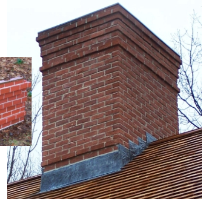
Above: Chimney mock-up used on job site. Right: Note detail pattern on new chimney
