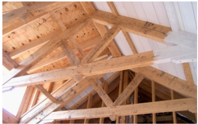
Partial finish work on ceilings is complete
