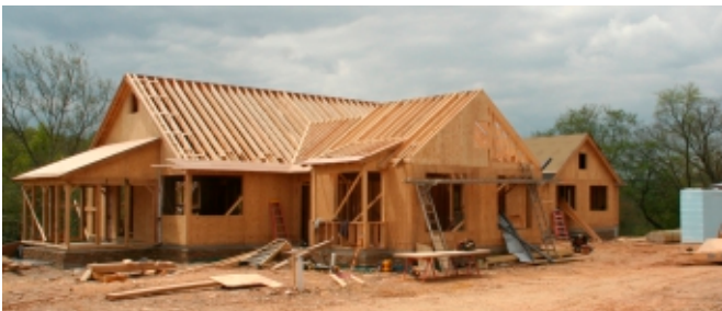
Framing work is well underway
