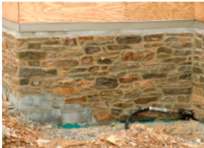
Natural stone siding will cover part of the walls, blending in perfectly with the natural surroundings
