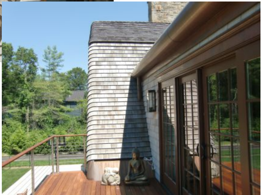
Unusual rolled eave finishing details were employed all over the roofline of the home.
